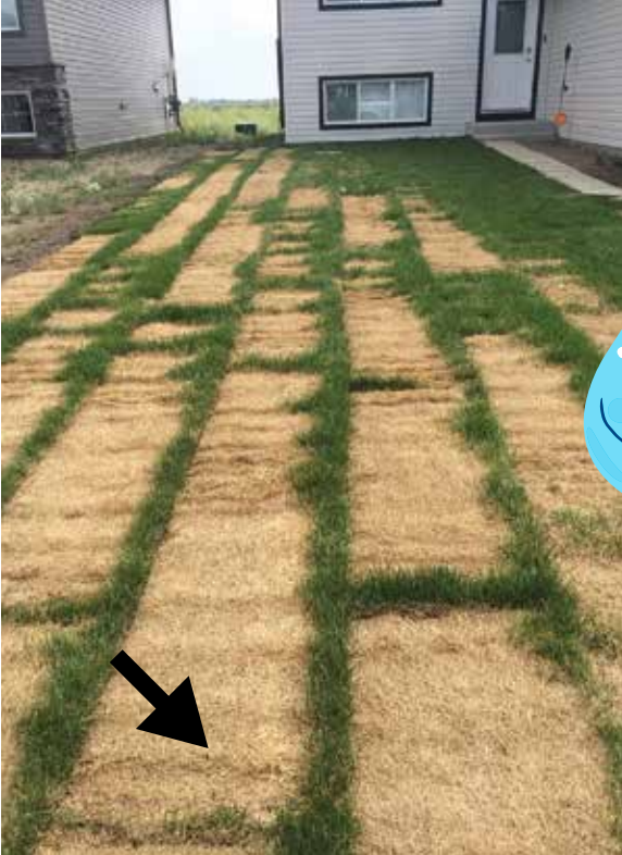
SOD THAT HAS NOT BEEN INSTALLED UPON DELIVERY.
